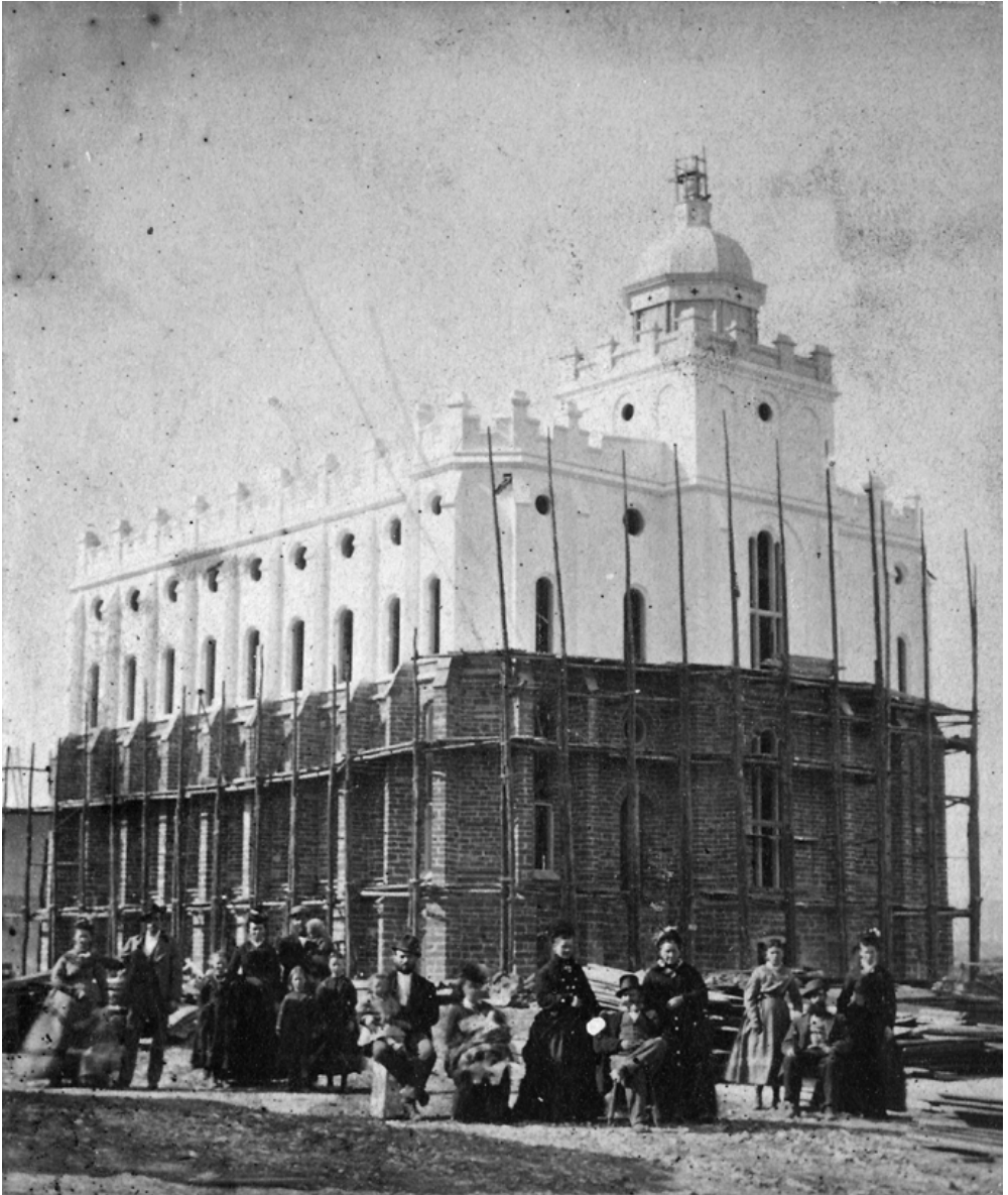
This view of the St. George Temple, ca. early 1876, shows the lower half of the sandstone being prepared for a whitewash coating, symbolizing purity and light. The main tower did not match Brigham Young's expectations; when it was damaged by lightning, it was replaced with a taller tower. This is the only known image of the temple under construction that includes a group of citizens in the foreground. Courtesy Harold B. Lee Library, Brigham Young University.
